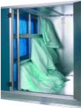
Panel/Bag Filter Section
